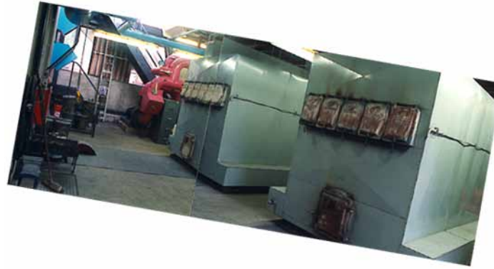
Boiler house or Plant Room at the Otago polytechnic, Dunedin, New Zealand - Location of the Plant Room installation
